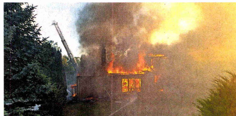
Two homes in Novi's Cedar Springs subdivision appear to be completely destroyed following a Saturday evening fire.
