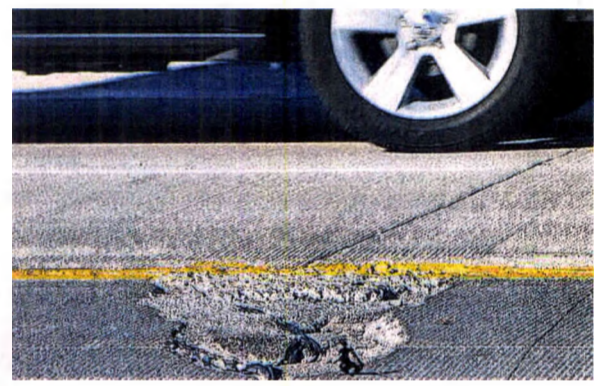
A pothole in the left-turn lane on Eight Mile. Wayne County says work to improve that lane will come later this year.
