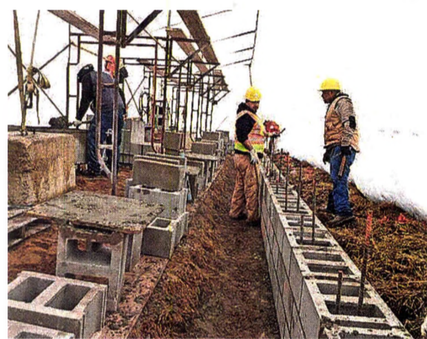
FILE PHOTO Early work on the new South Lyon Hotel is shown; the restaurant is expected to open in mid-August.
