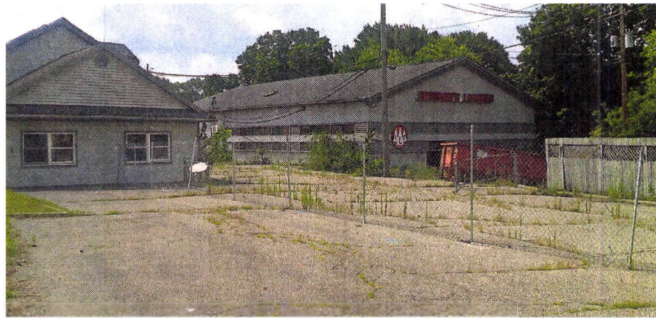
Buildings at the old Iverson's lumberyard await the wrecking ball.
