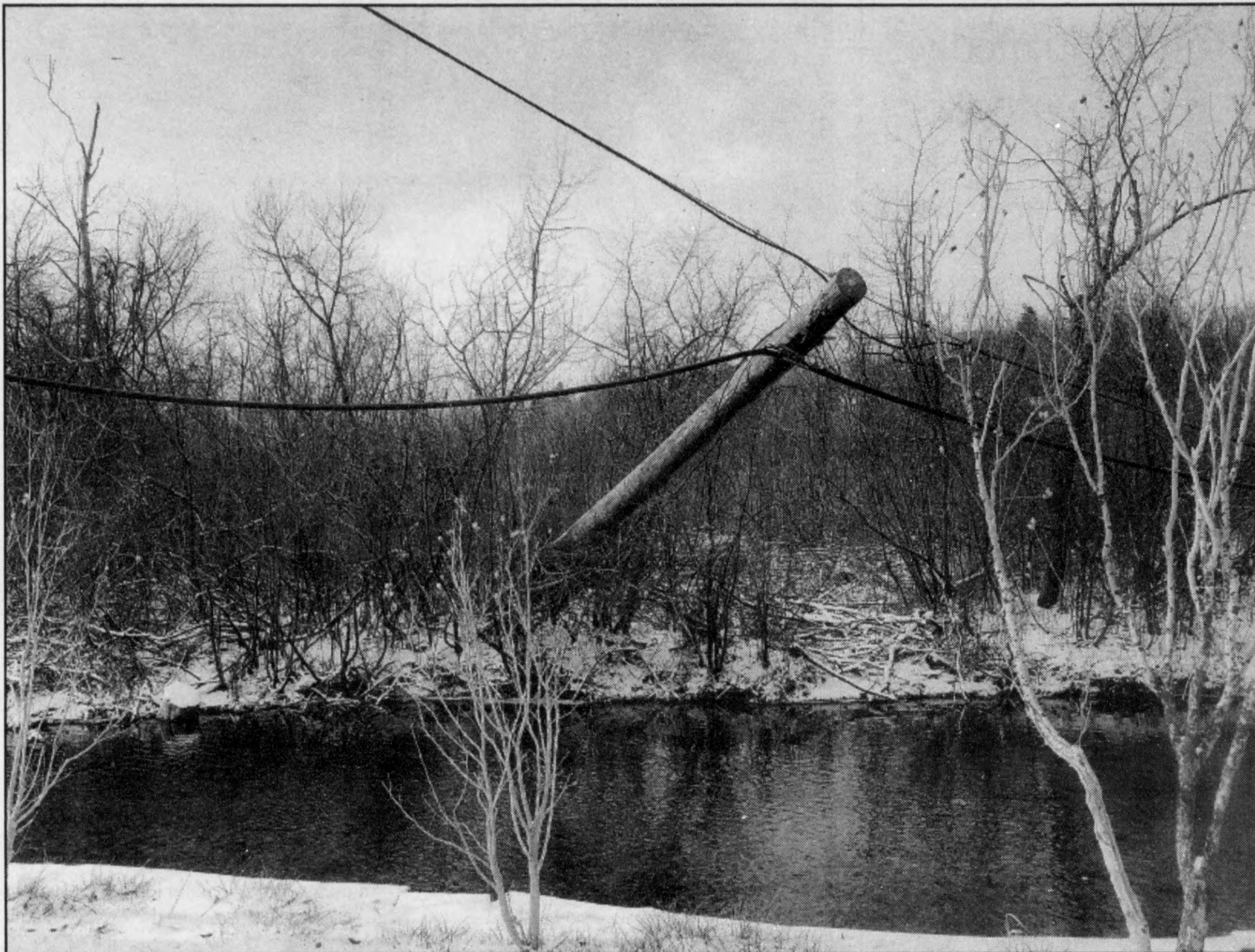
A broken utility pole leaves wires hanging over the water in the Clarkston park. Photo by Andrea Beaudoin
