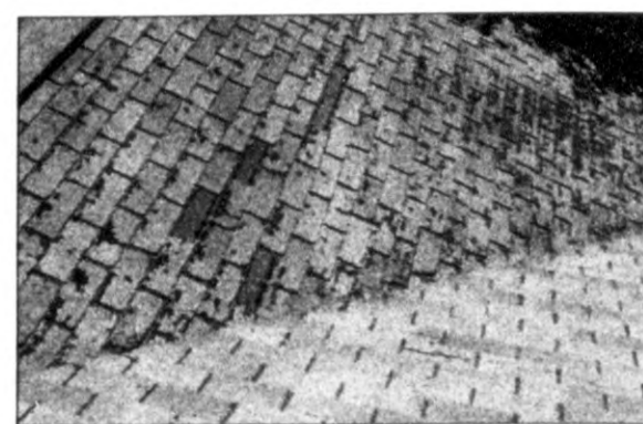
Lake Orion Roofing finds hail damage after inspecting the integrity of this homeowner's roof. Damaged shingles are not as effective in protecting the home from further leaks.
