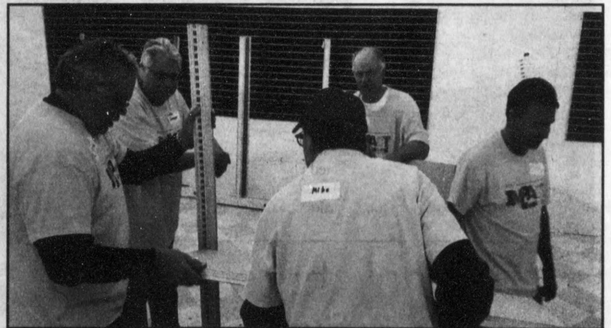
Volunteers can also work on indoor construction work. Photos provided
