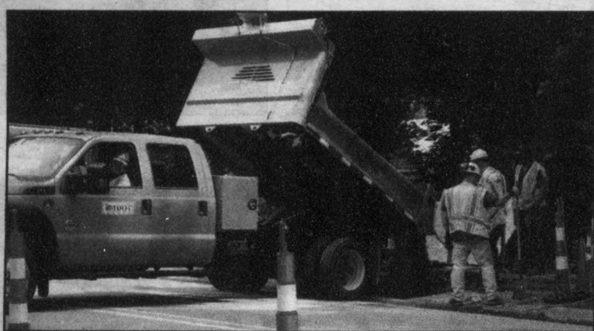
ROAD WORK: Michigan Department of Transportation workers fill a sinkhole at 20 N. Main Street after repairing a broken one-inch storm drain, June 15. The work is at no cost to the city, because M-15 is a state route. Clarkston City Council authorized the repair work north of Washington Street on May 29. Photo by Phil Custodio
