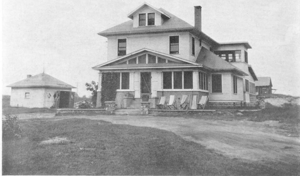
PRESENT T. B. HOSPITAL—OAKLAND AVENUE
