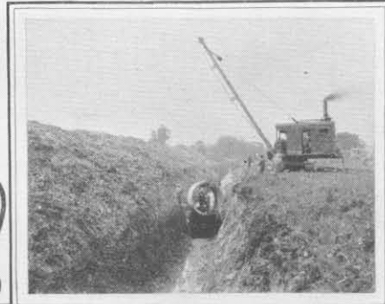
Placing 9foot pipe in position
