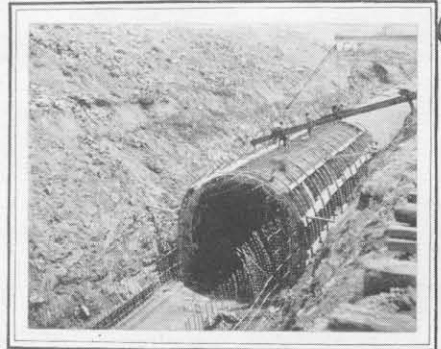
Reinforcing 15 foot pipe with Steel
