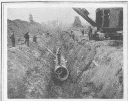
Laying 60inch Pipe
