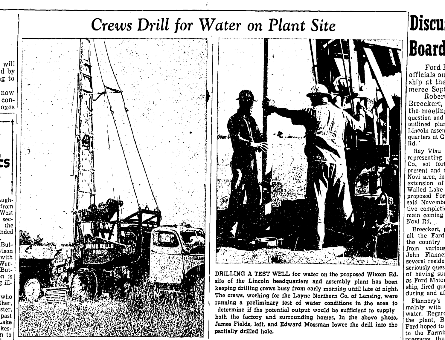
DRILLING A TEST WELL for water on the proposed Wiscom Rd. site of the Lincoln headquarters and assembly plant has been keeping drilling crews busy from early morning until late at night.
