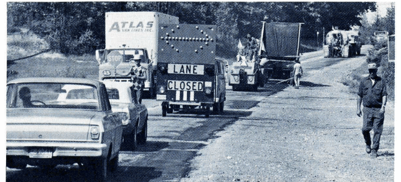
Repairing edge failure in an urban area.
