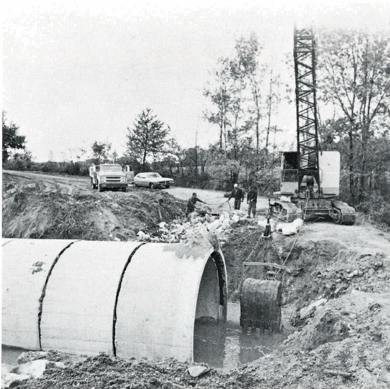
Maintenance forces replacing rural area bridge.
