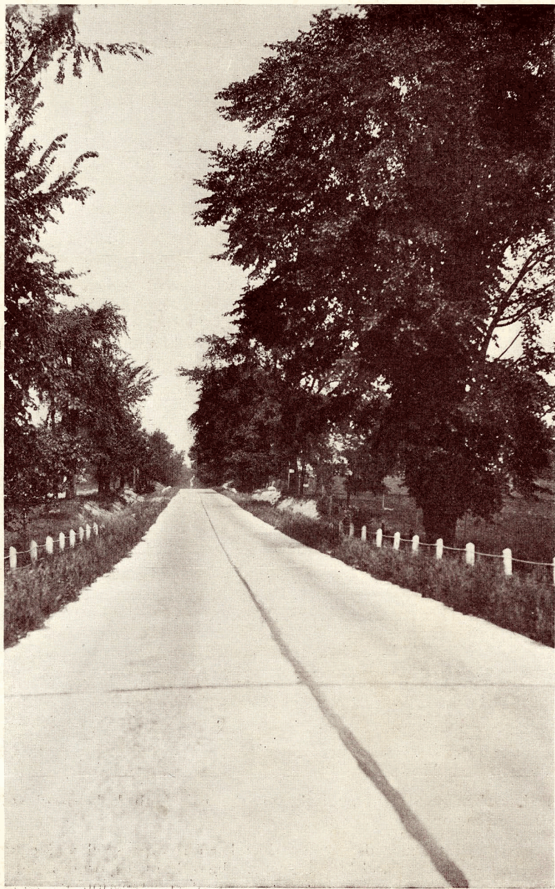
CASS LAKE ROAD (North)
