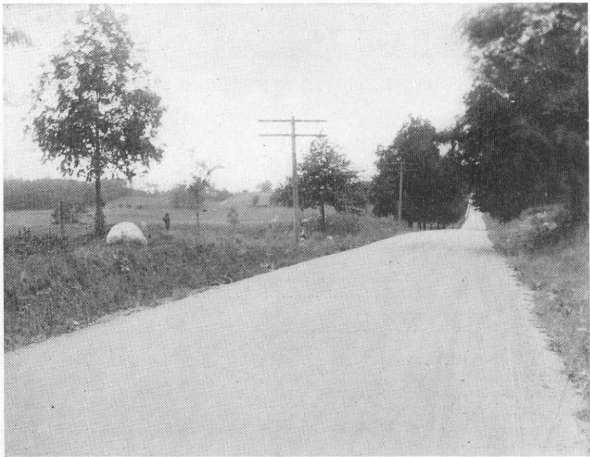
Constant maintenance keeps the Milford Gravel Road in good condition.
