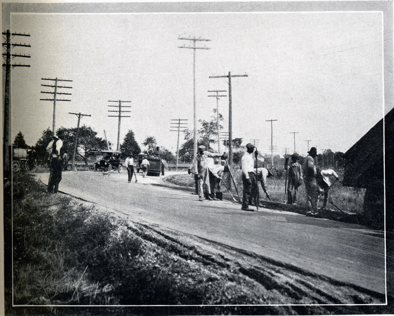
Asphalt crew repairing Oakland Avenue pavement
