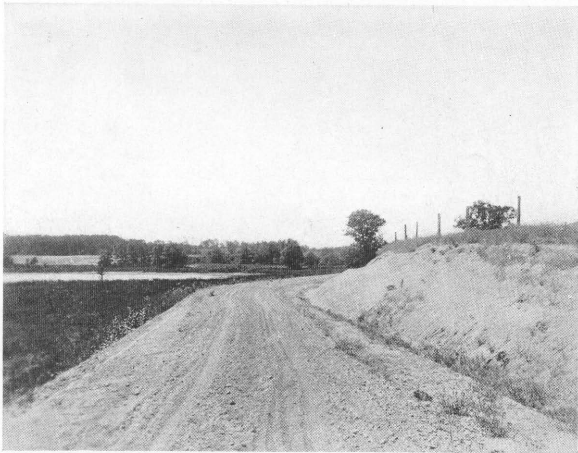
View on Davisburg Road, Springfield Township, showing terraced bank providing longer range of vision on what would otherwise be a dangerous turn.
