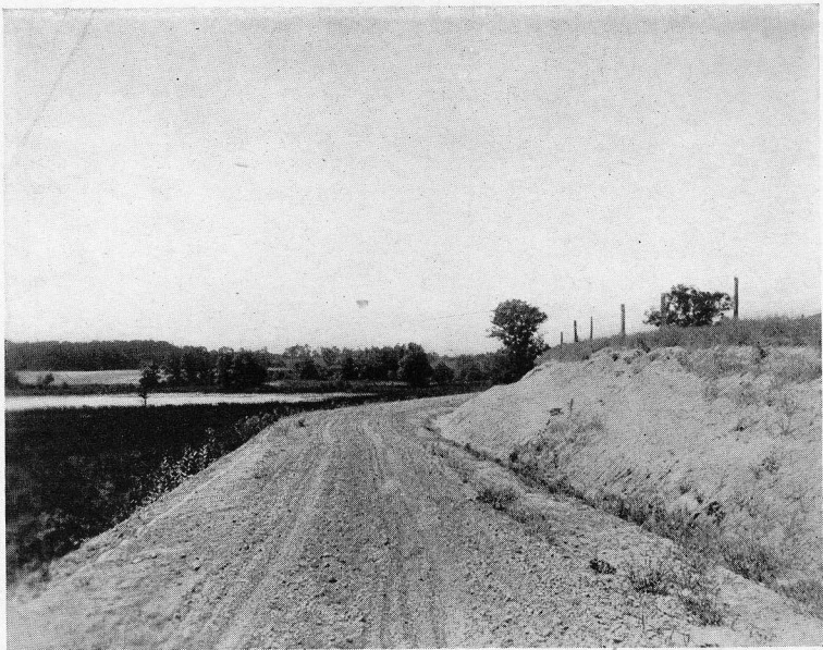
View on Davisburg Road, Springfield Township, showing terraced bank, providing longer range of vision on what would otherwise be a dangerous turn.
