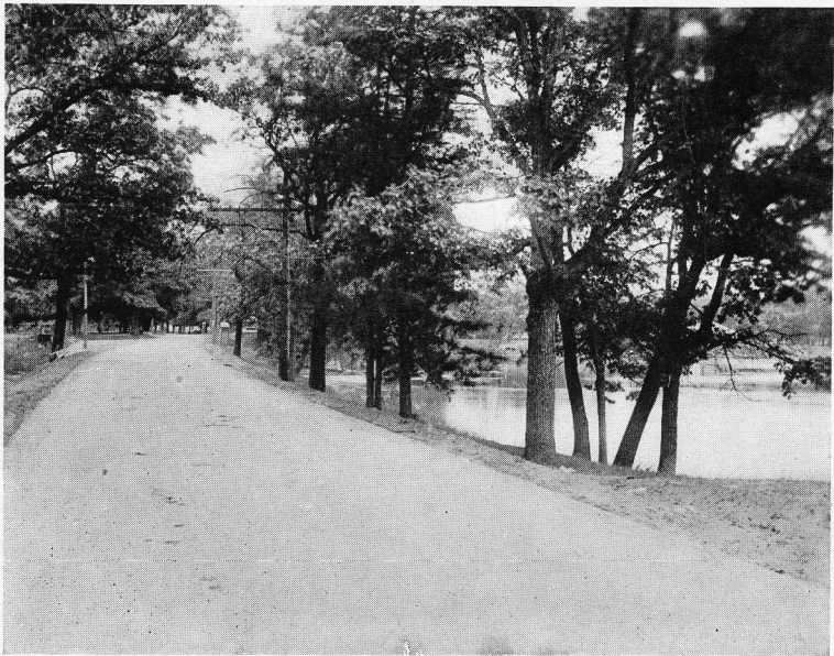
Concrete Paving on Orchard Lake Road.
