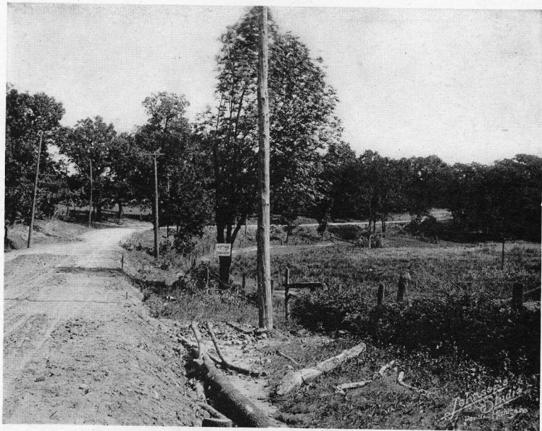
Gravel Road linking Commerce Gravel with Orchard Lake Concrete Pavement
