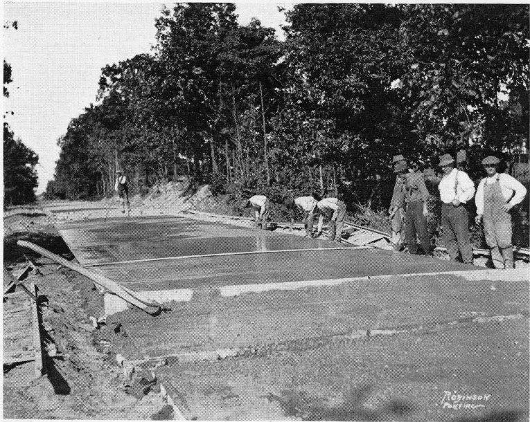
All stages of finishing surface of Concrete Pavement. Long Lake Road.
