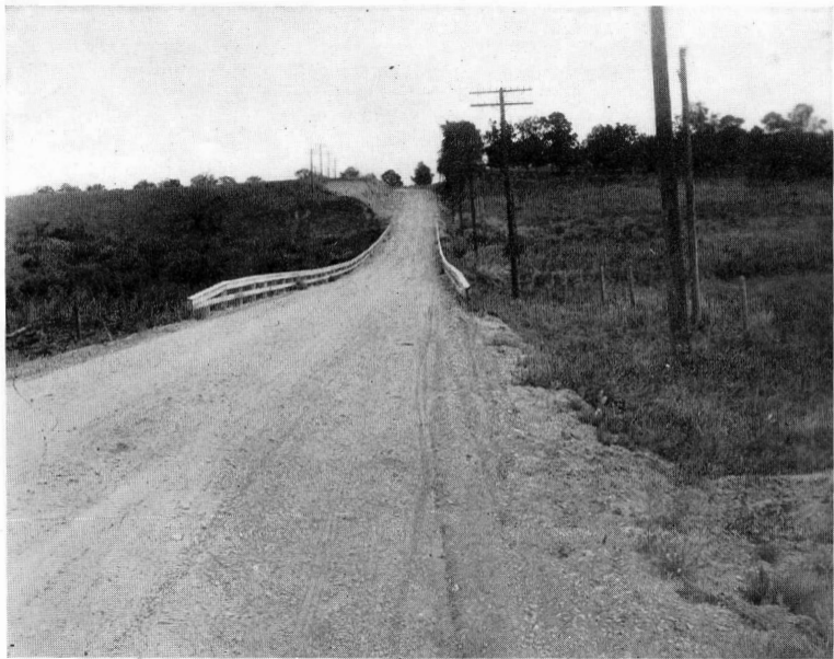
One of Oakland County's Sink-holes, on Saginaw Road in Holly Township.
