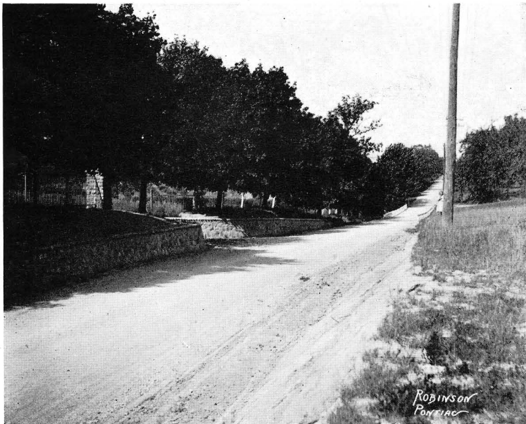
Stone Retaining Walls beautify the roadside. Dodge Road.
