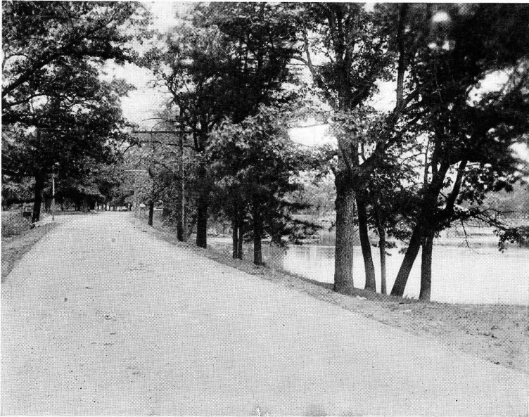
Concrete Paving on Orchard Lake Road.
