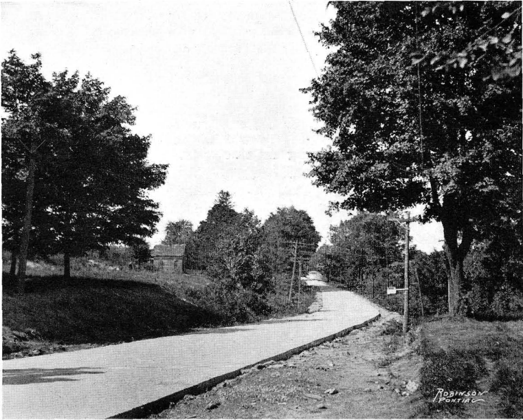
Concrete Pavement under construction. Milford Village.
