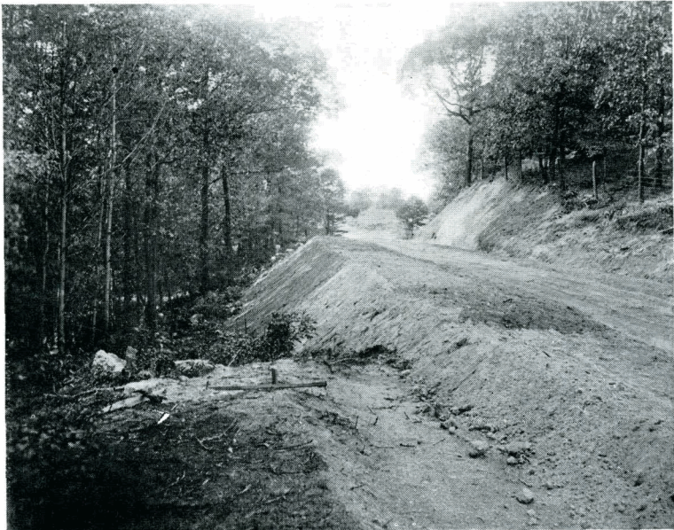
Scene on Elizabeth Lake Road. A difficult piece of construction.
