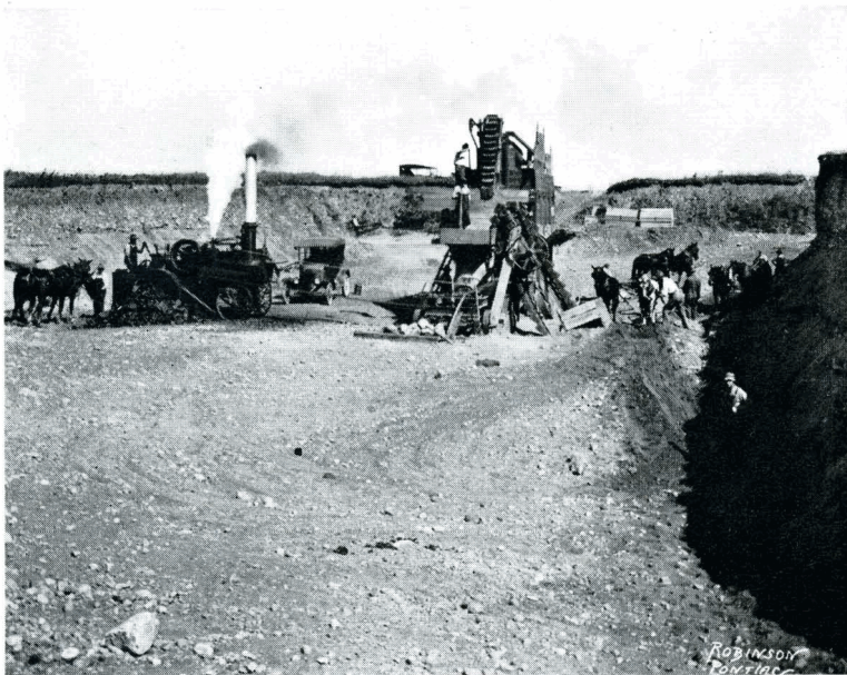
A Gravel Screening and Crushing Plant, County Pit. Highland Township.
