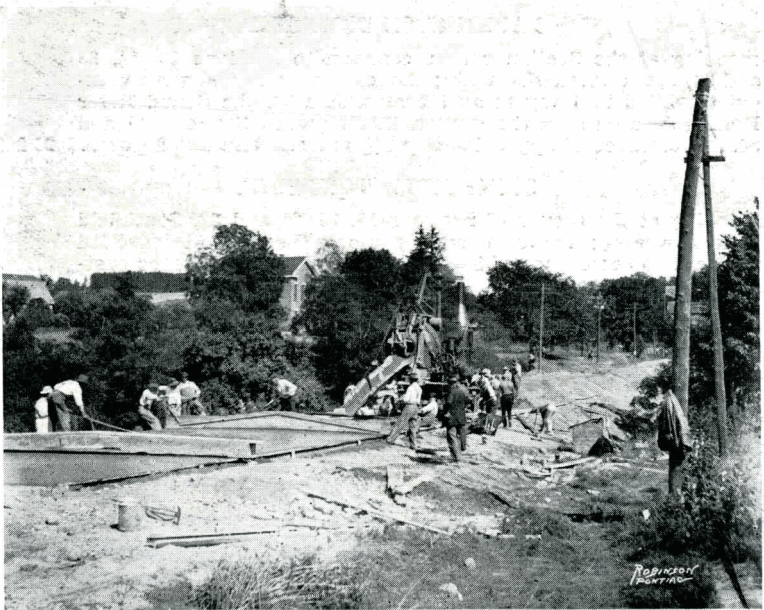
Paving Crew at Work. Material Dumped on Sub-grade, Milford Village.
