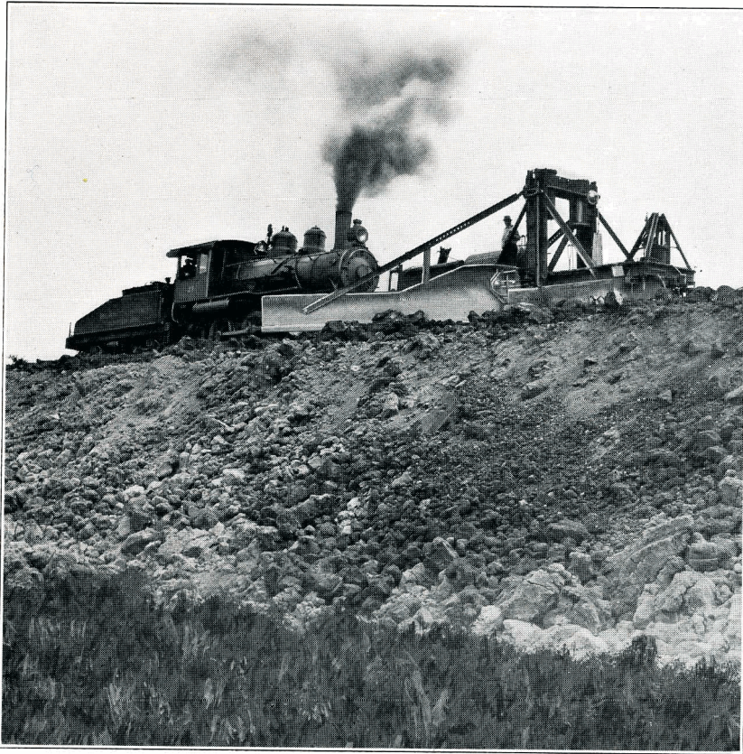
Modern Machine in Use in the Construction of Railway Grades
