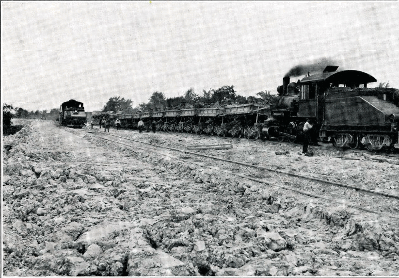
Trainloads of Fill Material Being Dumped in Embankments
