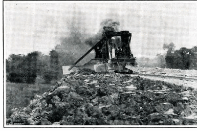
Leveling of Embankment
