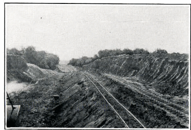
Temporary Track Used to Transport Filling Material
