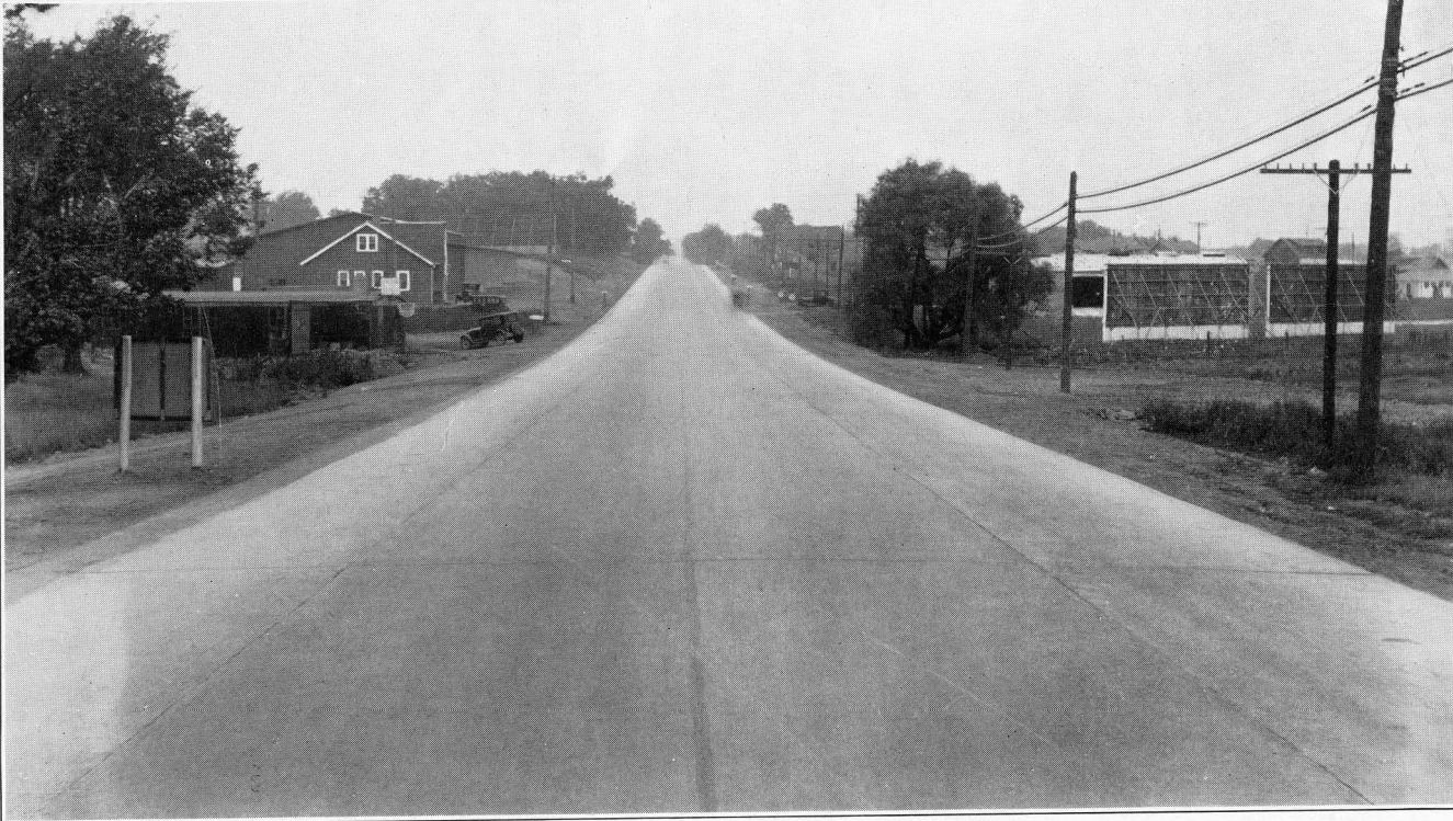
Concrete Road Widened to Forty Feet—Dixie Highway
