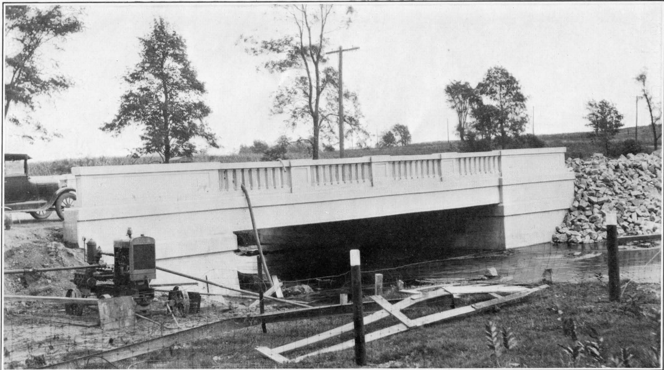
Ten Mile Road Bridge
