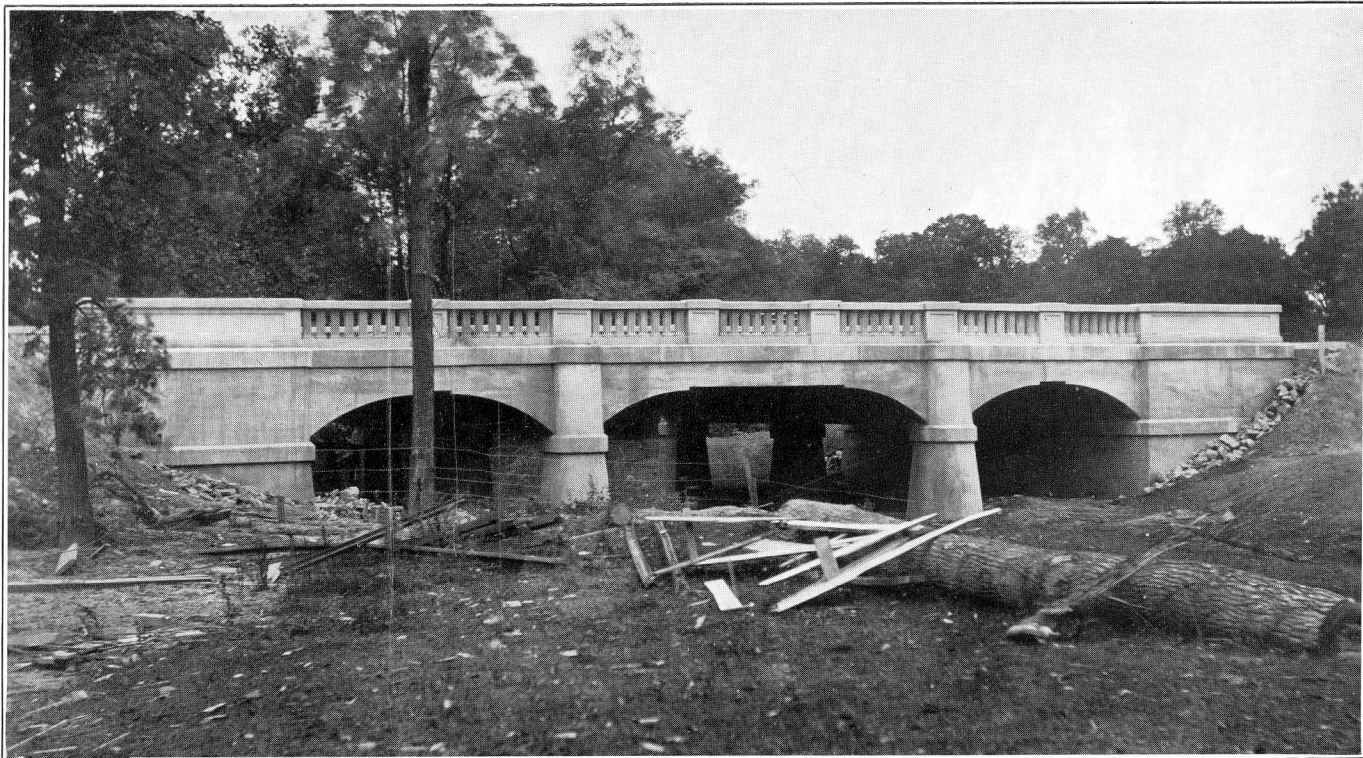
Ten Mile Road Bridge
