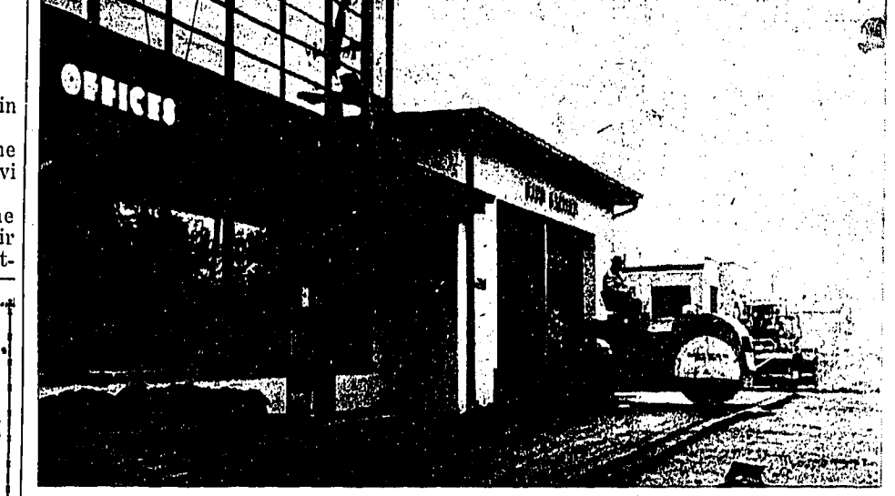
IF FIRST IMPRESSIONS COUNT, Novi Township officials will make a better impression on future visitors effective today. The summer dust and winter mud are now a thing of the past since the completion last night of the asphalt parking area in front of the office building. The Plymouth Paving Co. local contractors, did the work. One of their steam rollers is shown packing down a newly laid strip of asphalt.
