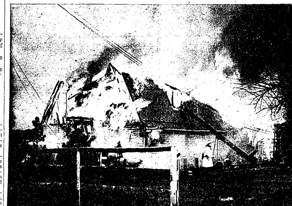
The roof fell in — and the walls came tumbling down. Fire flamed uncontrollably at the Northville Riding Academy last Friday and although several neighboring fire departments helped to fight the blaze, the situation became a hopeless one.
