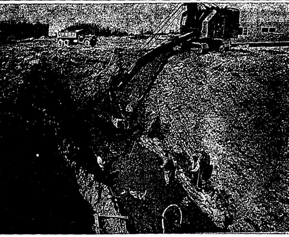
WORK IS PROCEEDING according to schedule at the site of the new Lincoln plant, according to company officials. Excavations are being made (above) for a sewerage disposal system to carry off waste from the painting operations in the new assembly plant. In the upper left is the C&O railroad spur entering the plant from the north. The long house trailer behind the power shovel is one of many such trailers on the site housing construction company offices.
