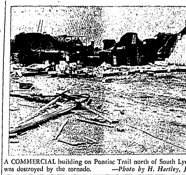
A COMMERCIAL building on Pontiac Trail north of South Lyon was destroyed by the tornado. —Photo by H. Hartley, Jr.
