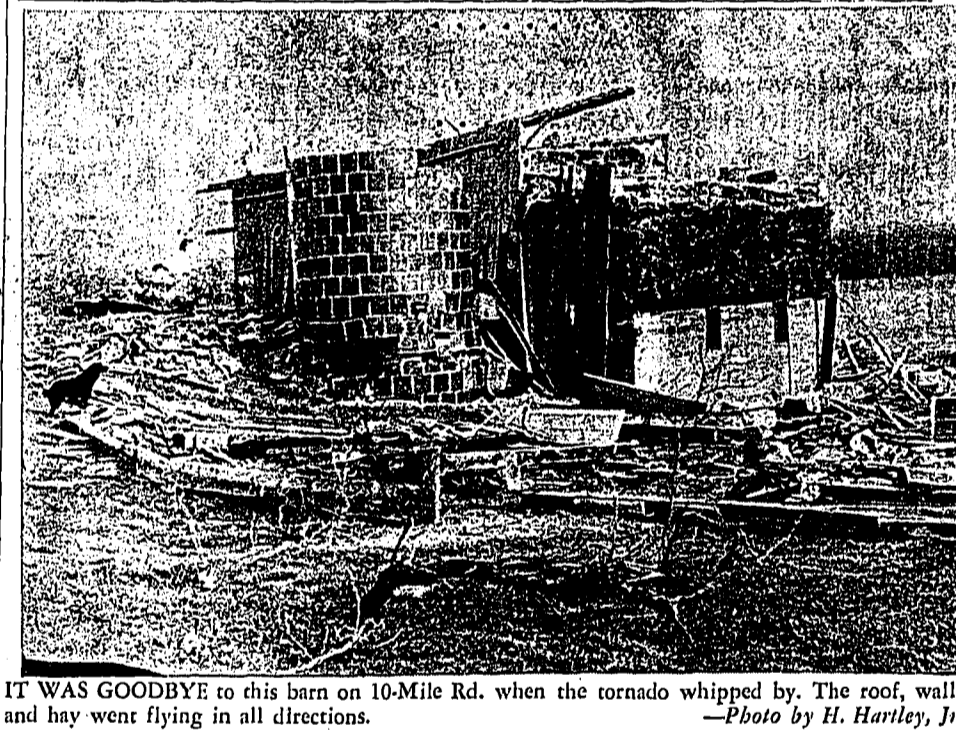
IT WAS GOODBYE to this barn on 10-Mile Rd. when the tornado whipped by. The roof, walls and hay went flying in all directions. —Photo by H. Hartley, Jr.
