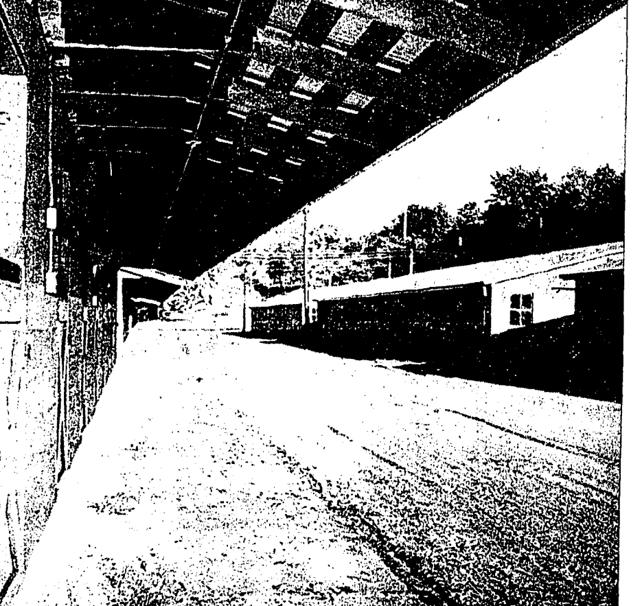
VACANT AT PRESENT, the new barns eventually may quarter horses year-round. The new complex includes three winter barns, nine summer barns, a utility shed, a blacksmith shop and a restaurant. All are fireproofed with concrete block and aluminum construction.
