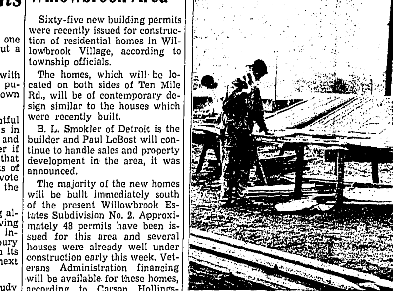
FABRICATING AND ASSEMBLING ROOF TRUSSES for new homes in Willowbrook will be well under way this week with announcement that approximately 65 new building permits had been granted to B. L. Smokler & Co., Detroit builders.
