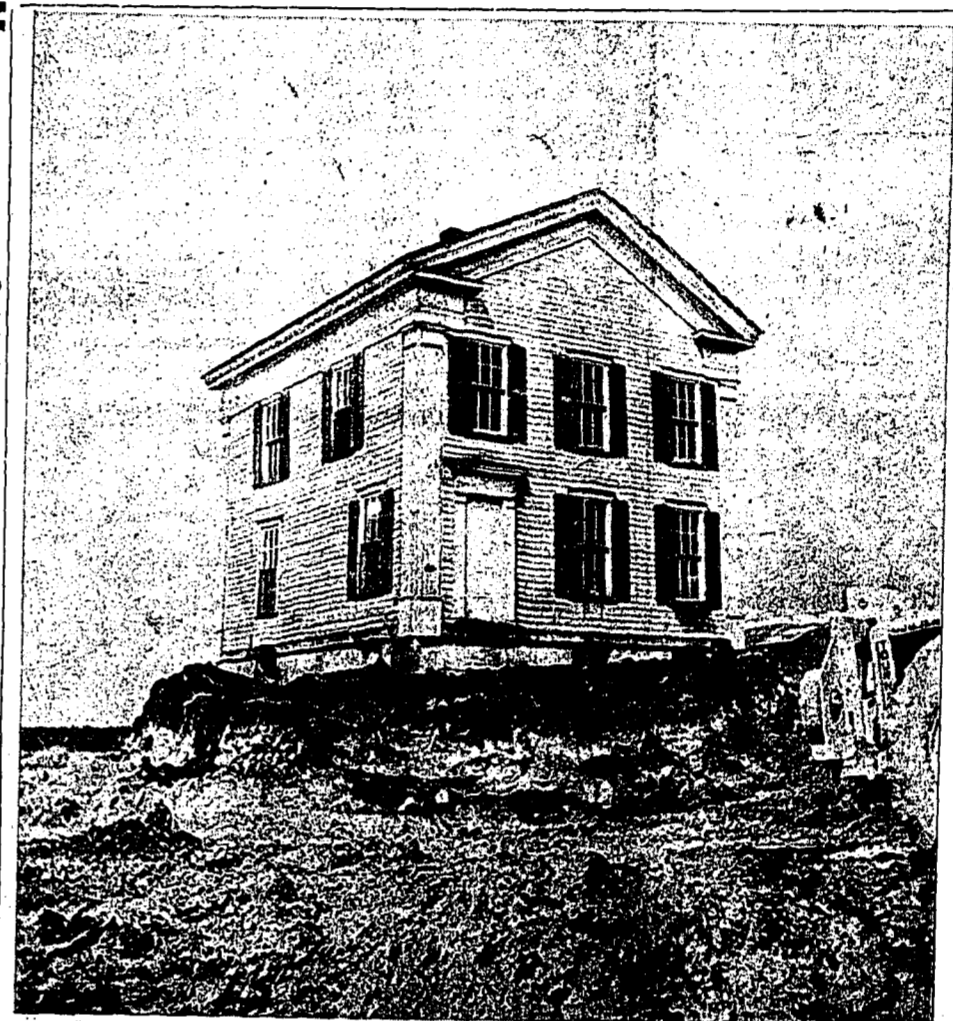
THIS OLD HOUSE, formerly owned by J. A. Applehof, is left high and dry as work progresses at the new Lincoln plant. Now being used as a field office for engineers and surveyors, the house is scheduled for eventual demolition.
