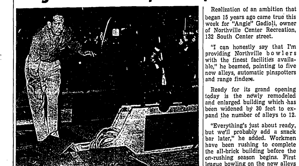
OWNER ANGELO GADOLI takes a close look at his new automatic pinspotters as they are being installed at Northville Center Recreation. "Angie" plans to open the newly remodeled 12-lane alleys today.
