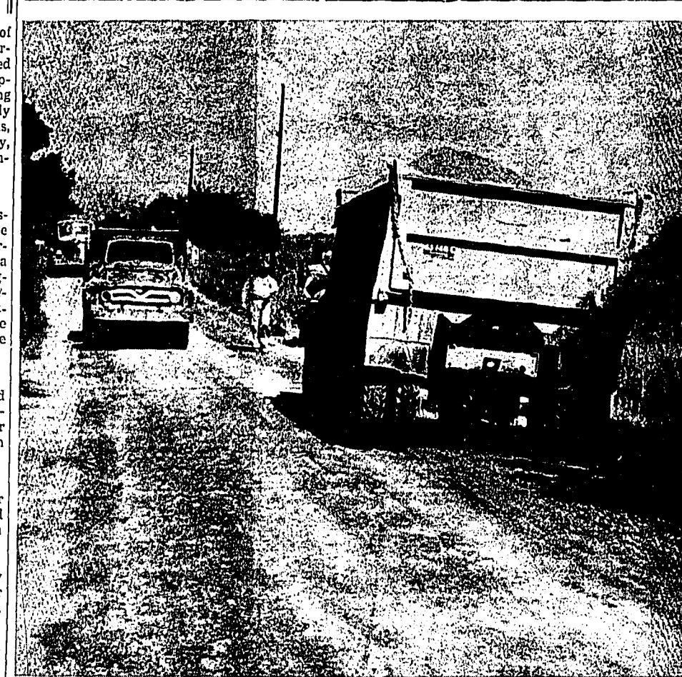
MECHANIZED HEADACHES — Residents of Taft road and other township roads feel that something should be done about these construction trucks that rumble past their homes on the way to and from the Brighton-Farmington expressway. But county road officials say the trucks must have an access to the site if the super highway is to be built.
