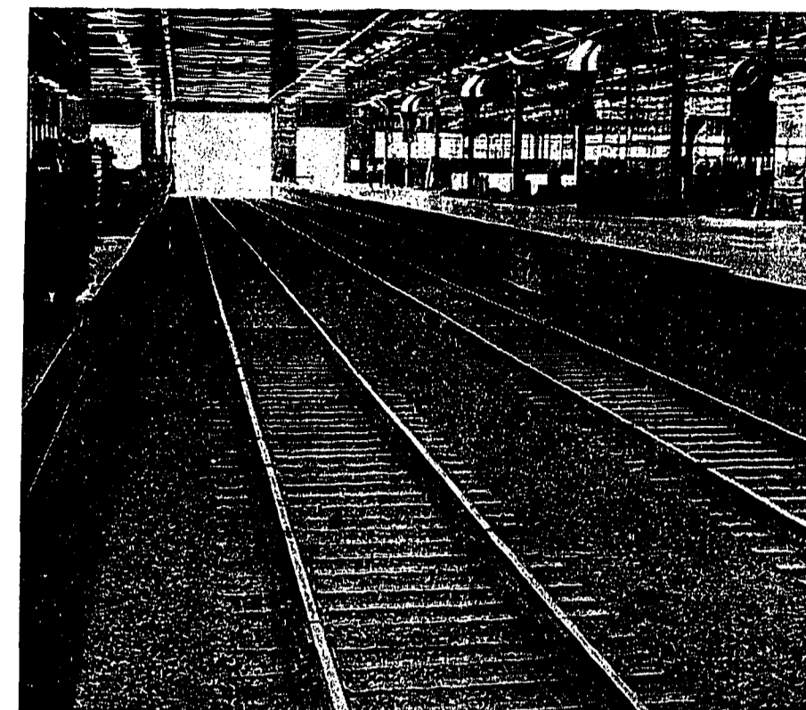
SOME 34 RAILROAD CARS can be accommodated simultaneously in the new Lincoln plant where 1,800 tons of materials will be unloaded daily. There are also facilities for handling 24 trucks. The tracks are located inside the plant in such manner that freight cars can enter or leave either end of the manufacturing building.
