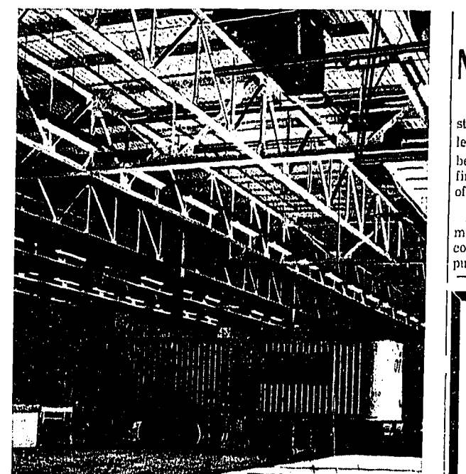
TRUCK DOCK AT THE NEW LINCOLN PLANT which opened this week is capable of holding 24 trucks at one time. The dock, coupled with a lengthy railroad track running inside the building from two ends, give the new plant complete facilities for handling the tons of material that come in daily.
