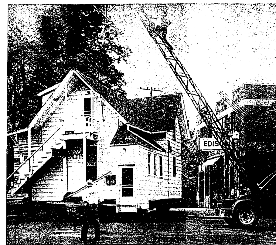
STARTING out on its trip to a new location, the house makes a careful turn at Center and Dunlap as workmen (top of picture) watches power line clearance.
