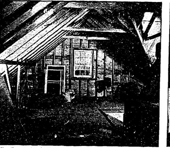
Like thousands of other expansion attics this was a good store . . . and a golden opportunity for the extra space the homeowner's growing family needs.
