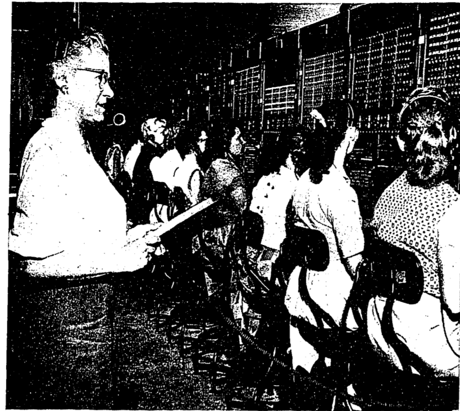
THE OLD manual-type switch-board will pass out of existence when dial service comes to Northville early Sunday. Mrs. Lillian N. Timm of Oak Park, chief operator here for Michigan Bell Telephone Company, is shown supervising some of the final calls made over equipment in the old telephone building.
