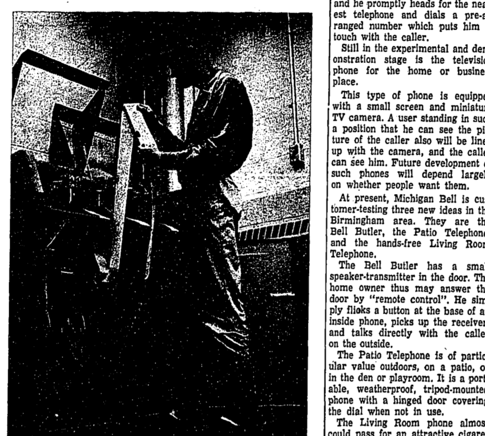
AUTOMATIC MESSAGE ACCOUNTING equipment goes into operation along with Northville's new dial system. Here, Chester Sandek, a Western Electric installer, reads the tape which records billing information such as the calling telephone number, the party dialed, and length of call.
