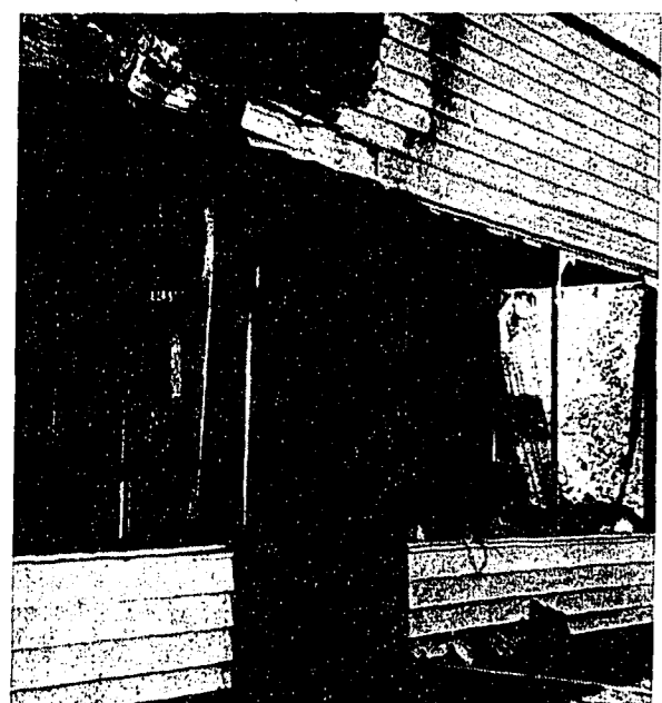
GUTTED —A flash fire broke out last Wednesday night at the printing plant in Plymouth of Glen Cummings, former Record-News publisher. Plymouth firemen fought the blaze but it had too much of a start. Equipment and supplies were badly damaged or destroyed. Cummings plans to rebuild soon.
