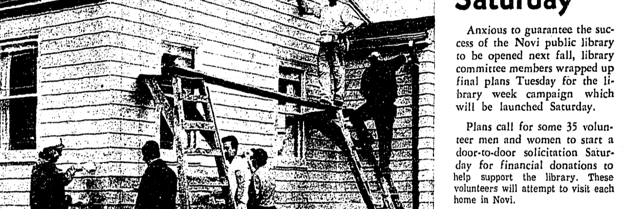
PAINTING BEE — Members of the West Shore Community Association finished in last week to paint the Novi public library building which will be opened for the first time next fall. The two-week job took the enthusiastic members only two evenings to complete—although rain forced postponement several days.
