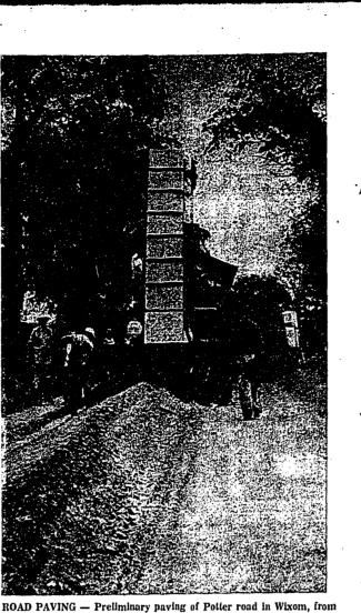
Wixom road to Beck, has been completed. The paving process, termed stabilization, consists of mixing road sand and gravel with asphalt. Cost of the project, part of a 10-year, \$200,000 road program, has been
