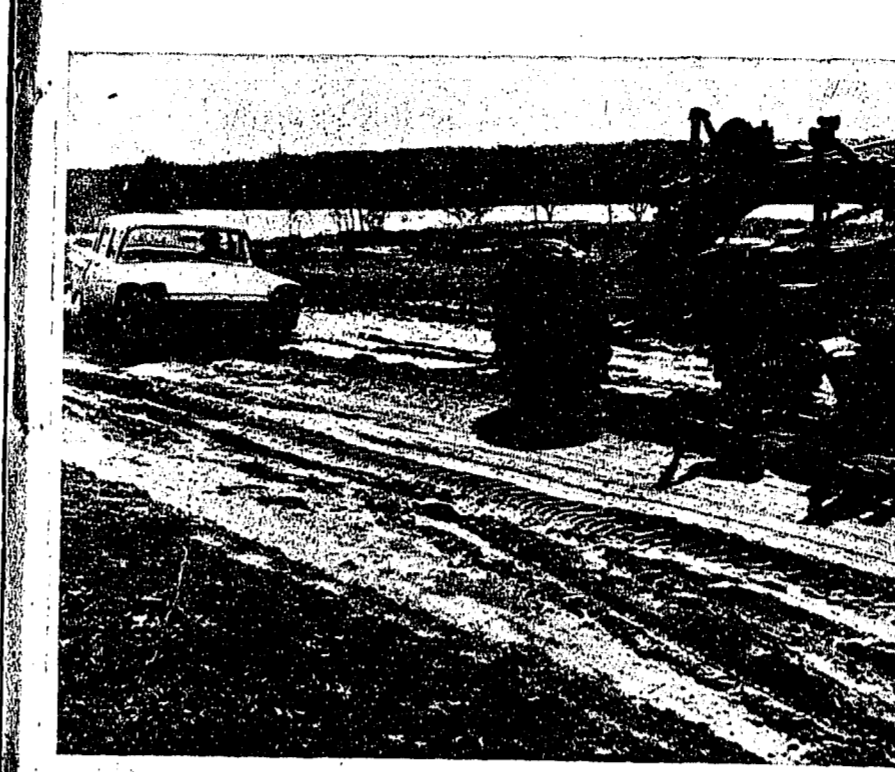
LOON LAKE ROAD, pictured above, drew criticism at the Wilson city council meeting last Thursday as residents complained about the "near-impassability" of the road. Here, the city's road grader is used to pull a molester from deep mud atop Hopkins hill. Salt used during the winter to keep the hill navigable after ice storms has drawn the frost from the road.
