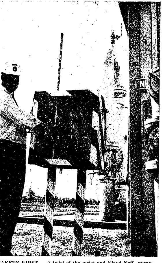
SAFETY FIRST — A twist of the wrist and Floyd Neff, pumping station superintendent, could shut down Consumers Power company's Northville station. The valve he's holding closes off incoming and outgoing pipe lines, shuts down the giant engines and compressors, disconnects the main power line and emergency generator and opens a blow-out valve to clear all pipes in the station. All operations except the blow-out require only 15 seconds. The blow-out would be completed within four to five minutes. Consumers has five such emergency stations located in its pumping facility. They would be used in case of a ruptured line, fire or other danger that could cause an explosion.
