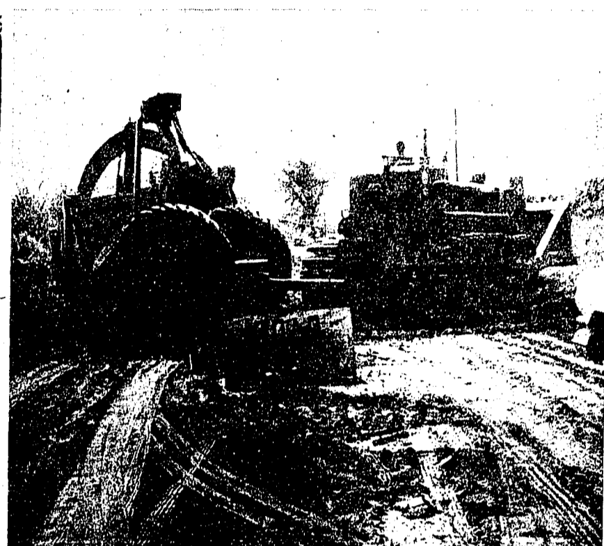
NORTH CENTER STREET, next in Northville's summer paving program, was being readied this week. After pulling trees and stumps, as above, workers began grading. Paving is expected to begin next week.
