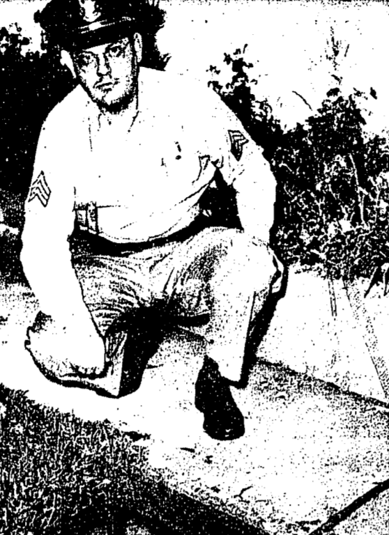
WHAT HAPPENED? - When Northville Police Sergeant Frank Heints returned to his Carpenter street home Saturday morning after eight days he found a three-foot deep hole under his back yard sidewalk. The earth had simply "sunk". Heints is puzzled as to the cause. No water or gas lines are in the area.
