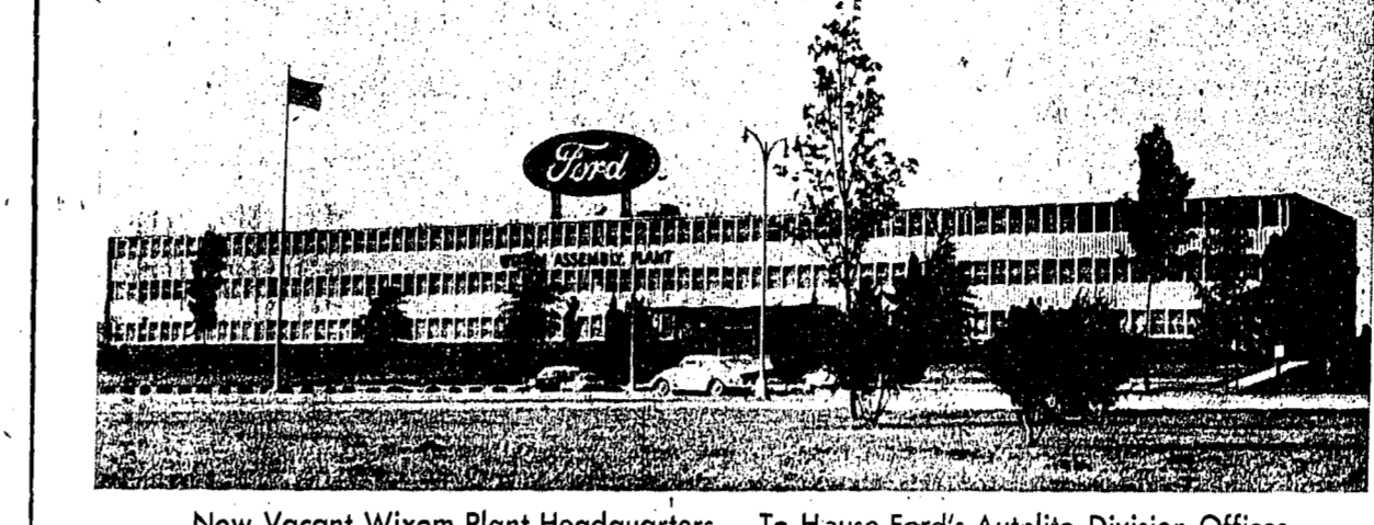
Now Vacant Wixom Plant Headquarters - To House Ford's Autolite Division Offices
