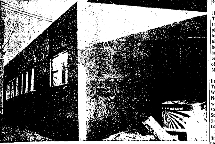
WELL UNDERWAY is the addition to the Novi community building, a 15 by 31 feet storage room with a 10' long vestibule being constructed on the north end of the building. Contractor Paul Palmer of Northville, who is building the $3,900 addition, said all work except roofing and interior finishing has been done. He said the job would be completed soon after delivery of roofing materials is made.
