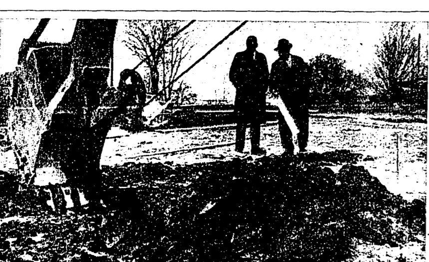
CONSTRUCTION BEGINS — A power shovel bit into the earth early Monday as construction of the long-awaited Salem school was launched. The new school is expected to be completed by fall. Watching the work are Architect James Madison and Contractor Paul Wallace.
