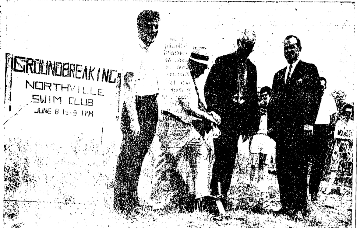
DIGGING FOR WATER — Mayor A. M. Allen and Township Treasurer A. M. Lawrence joined together to turn the first shovel of earth Saturday for construction of the Northville Swim Club's new pool and bath house. In the future a diving bay is planned, as well as an enlarged bath house and tennis courts.
