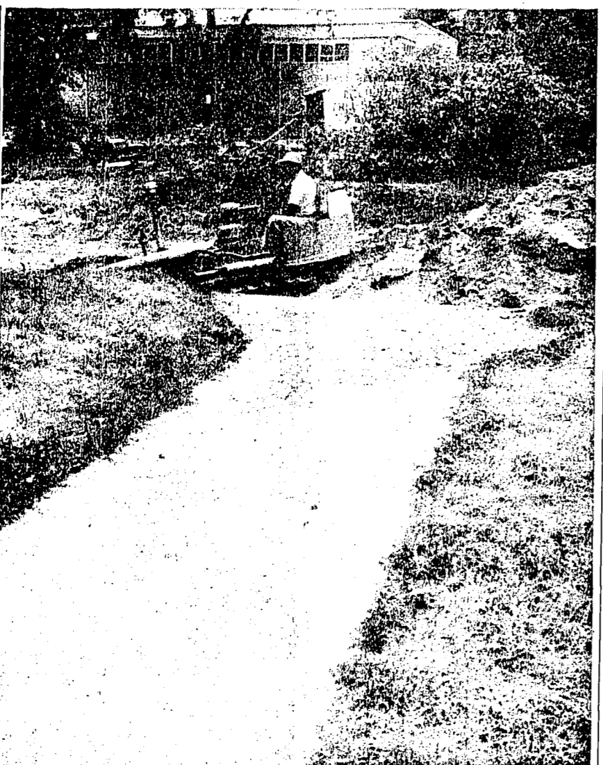
WATCH THAT FIRST STEP - The sidewalk that once led to the entrance of old city hall now comes to an abrupt end. Grading and tree removal is now underway preparatory to construction of the city's new $260,000 city hall-library. Contractors are hoping for completion by Christmas.
